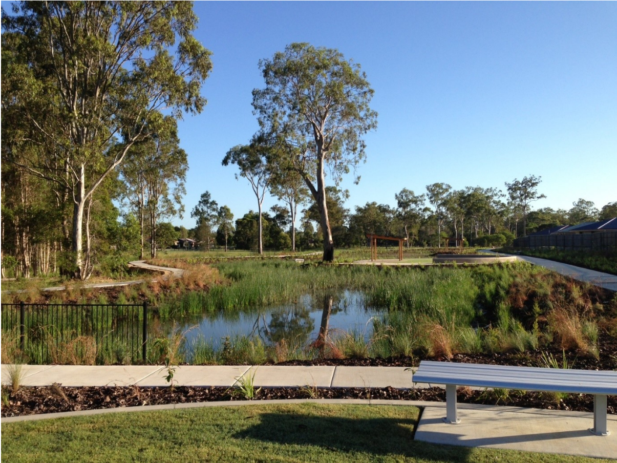
Figure 9.4.12. Photo of a Typical Constructed Wetland (Source: Steve Roso)
